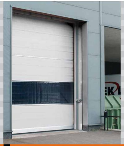
An exterior door should be left open for the shortest possible period of time. A traditional exterior door opens and closes relatively slowly, leading to considerable energy loss. However, energy loss can be minimised by combining a 'slow' exterior door with a high speed door.
